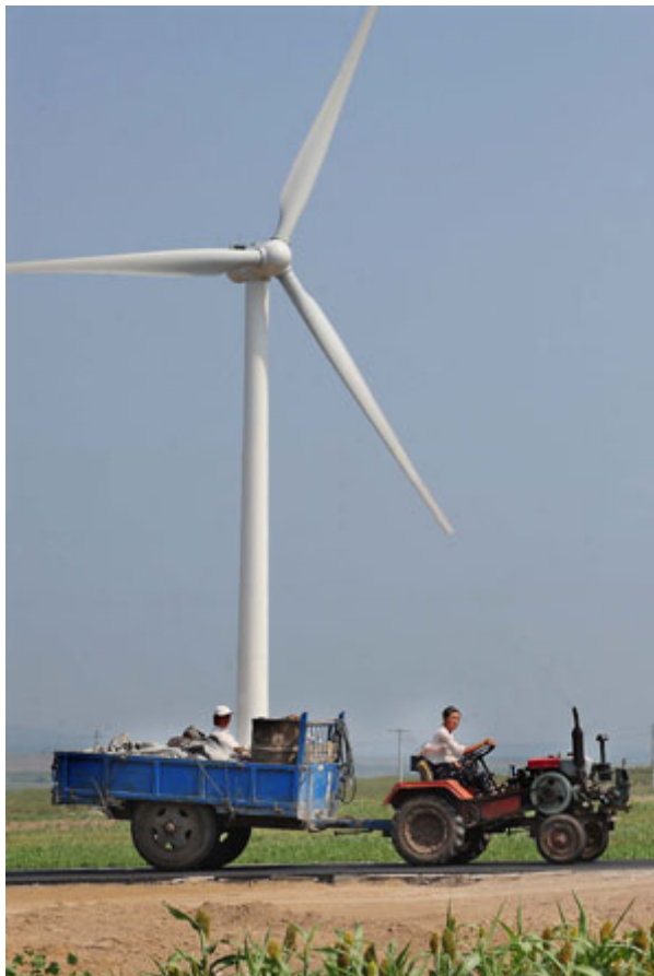
Wind turbines in Hinggan prefecture, Inner Mongolia
