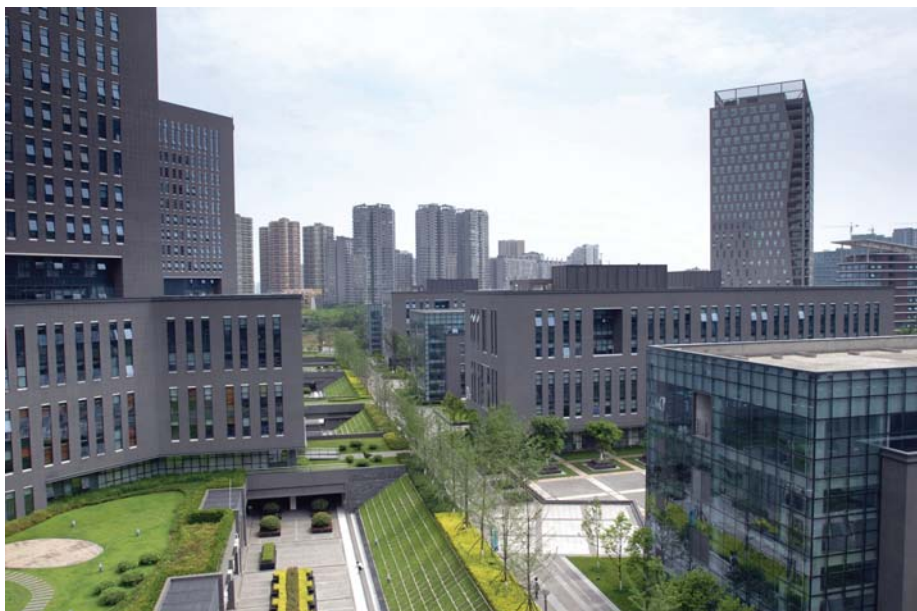
Commerical developments at the Tianfu Software Park in Chengdu’s Hi-Tech Industrial Development Zone.
